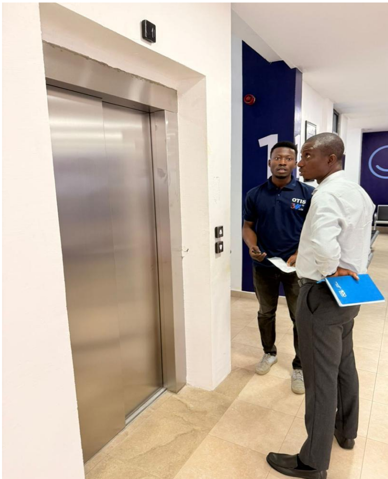
GHANA CLEFT FOUNDATION, KOMFO ANOKYE TEACHING HOSPITAL (KATH), KUMASI – INSTALLATION OF PASSENGER ELEVATOR
