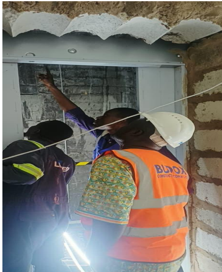
NATIONAL INSURANCE AUTHORITY (NHIA), LEKMA, ACCRA – INSTALLATION OF PASSENGER ELEVATORS
